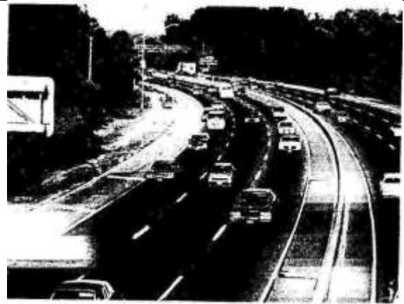
Level of Service B
